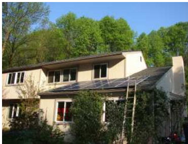
Suburban Home With Solar & Geothermal 1
